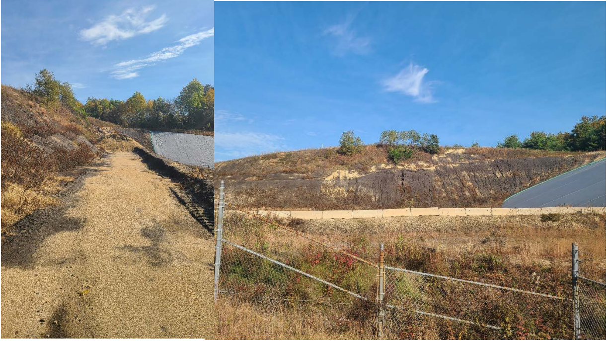
Photo 1: Active cell of the landfill with steep slope at working face looking north (right photo) from leachate collection building and east from east side of active cell (left photo)
