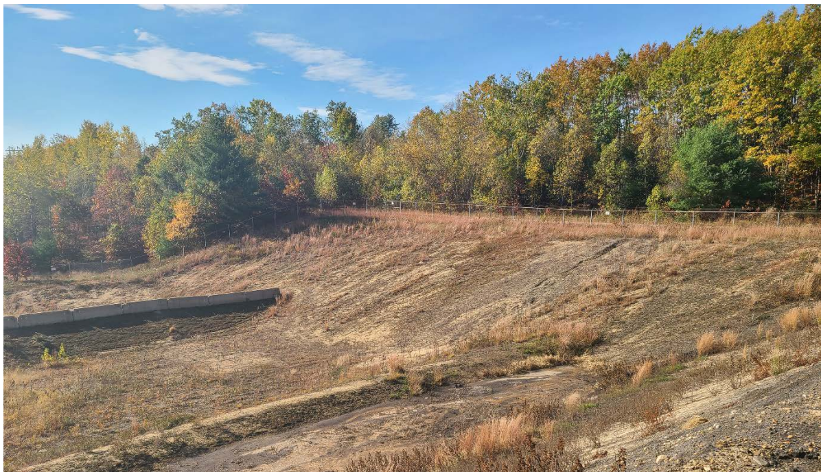
Photo 4: Landfill cells not currently in use looking southwest from southeast side of active cell.
