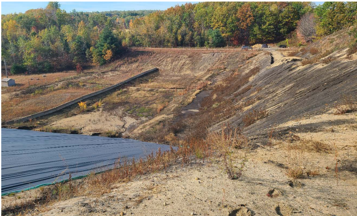
Photo 2: Active cell of the landfill with steep slope at working face looking west.
