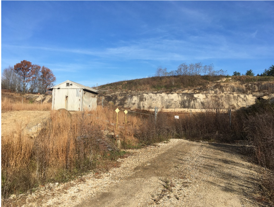
Photo 1: Landfill working face in the background and leachate collection building in foreground. The photograph was taken looking north.
