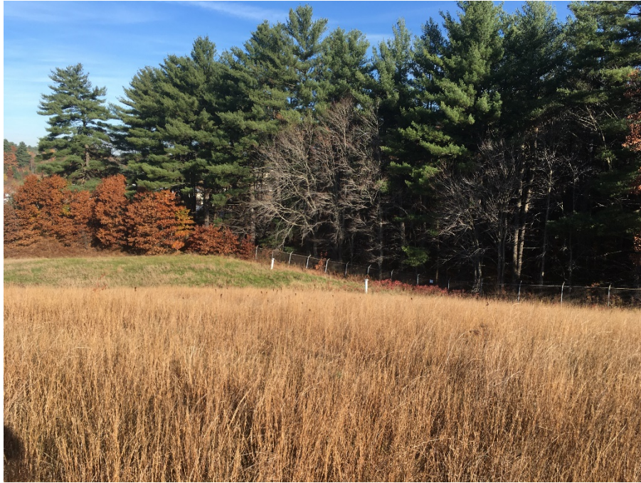
Photo 3: Stable and established slopes in inactive, capped area of landfill. The photograph was taken from near the top of the filled area and looking north.
