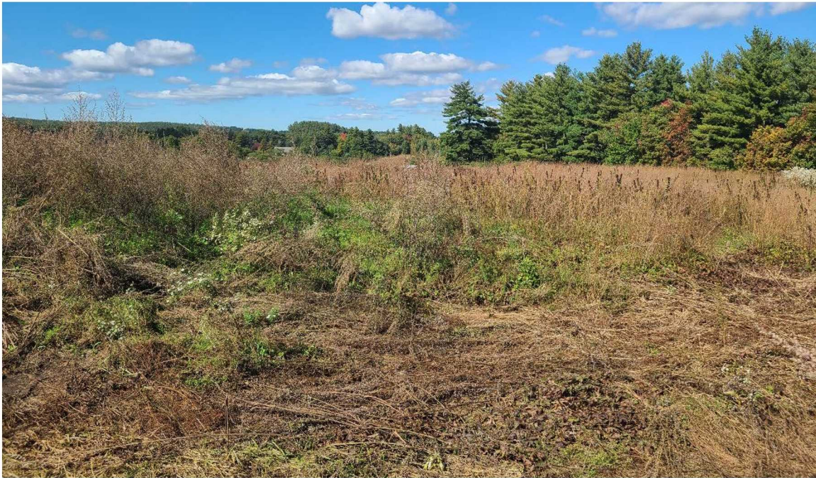
Photo 3: Stable and established slopes in inactive capped area of landfill looking north from top of filled area.
