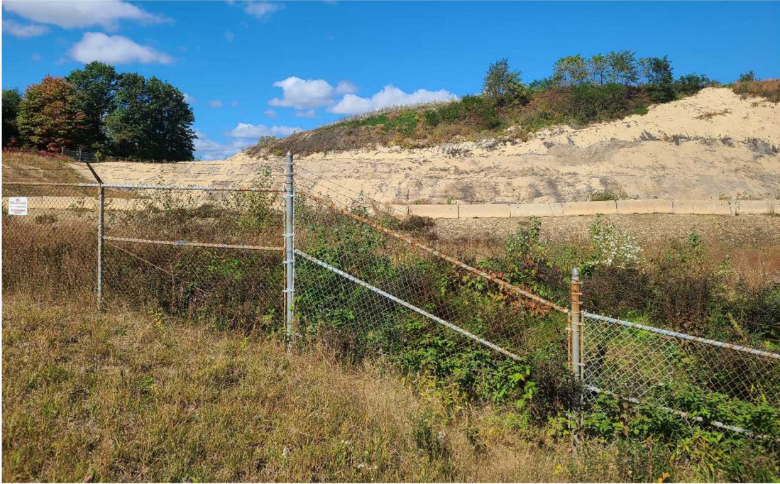
Photo 1: Active cell of the landfill with reduced steep slope at working face looking north from leachate collection building.
