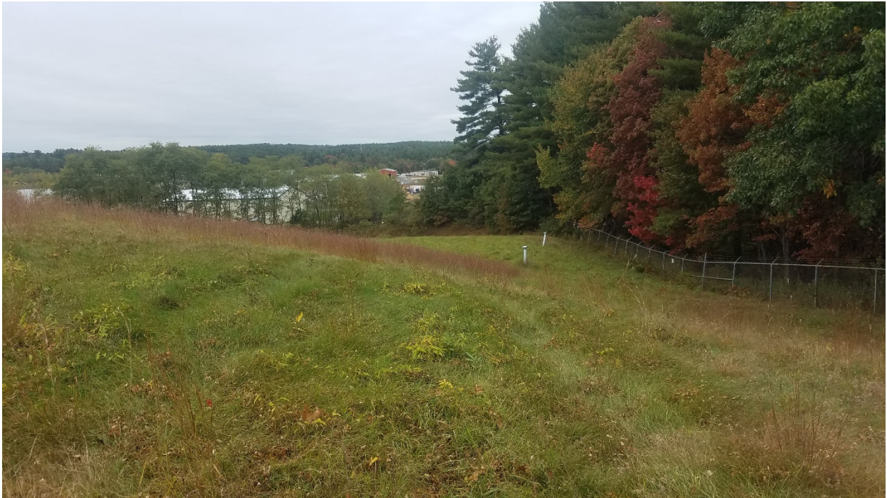
Photo 3: Stable and established slopes in inactive capped area of landfill looking north from top of active cell.
