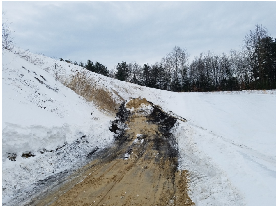
Photo 2: Active cell of the landfill with steep slope at working face.
