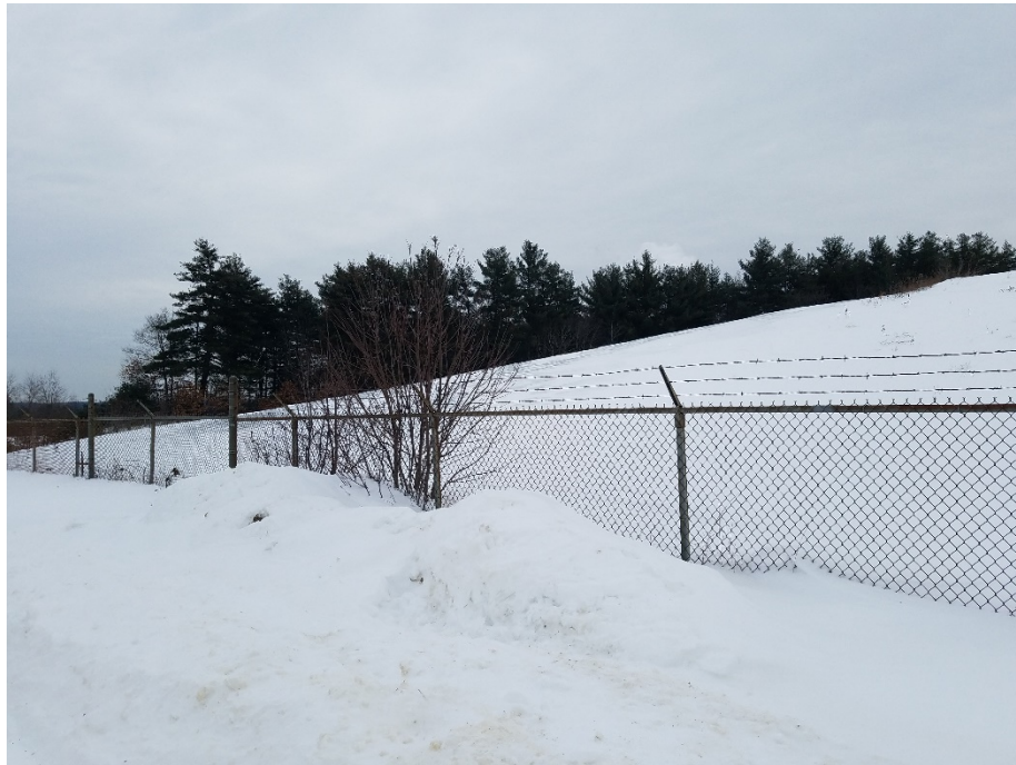
Photo 3: Stable and established slopes in inactive capped area of landfill.
