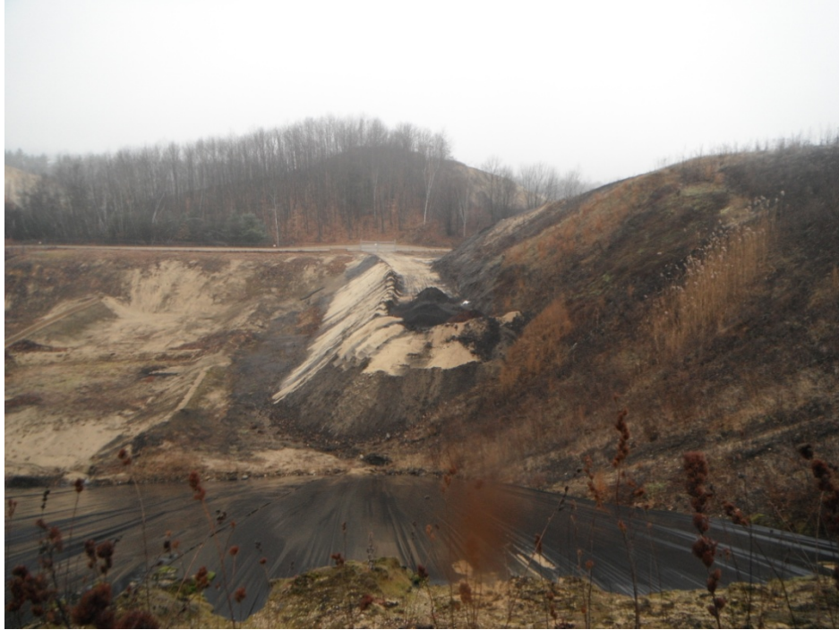
Photo 1: Active cell of the landfill with steep slope at working face.
