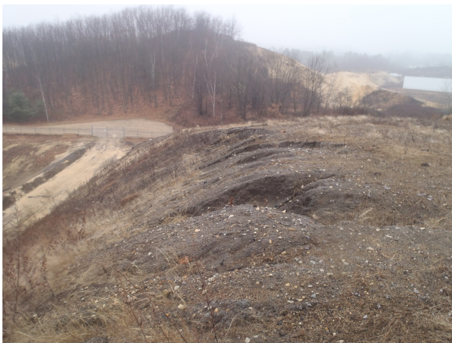
Photo 4: Limited erosion near active face of the landfill.
